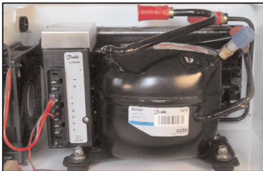
BD compressor with cover removed
